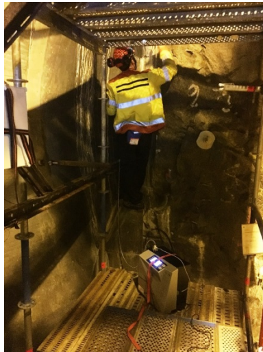
Helium sniffer leak search in June 2017. No track of gas could be detected on the downstream side of the dome!
