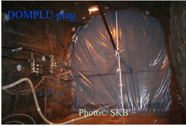
FSS swelling clay core emplacement
