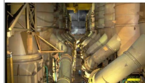
George Besse facility (France)
