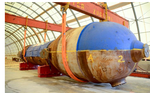
Disposal of a vapour generator at French surface disposal centre for VLLW (CIRES)
